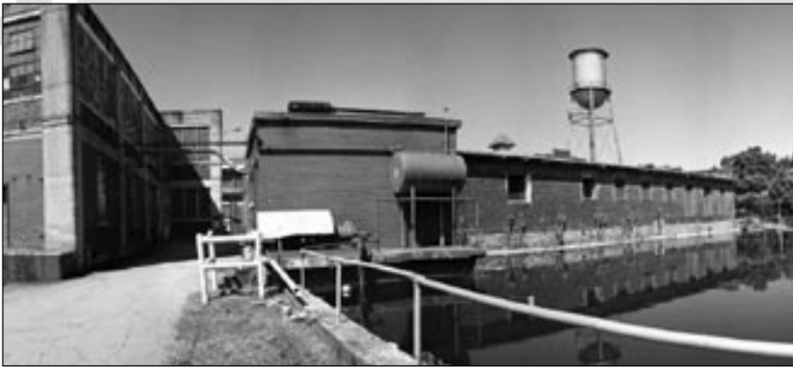
Photo: Exterior shot of mill buildings and reservoir.
